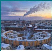
CM2023-06: Heating and cooling technologies
